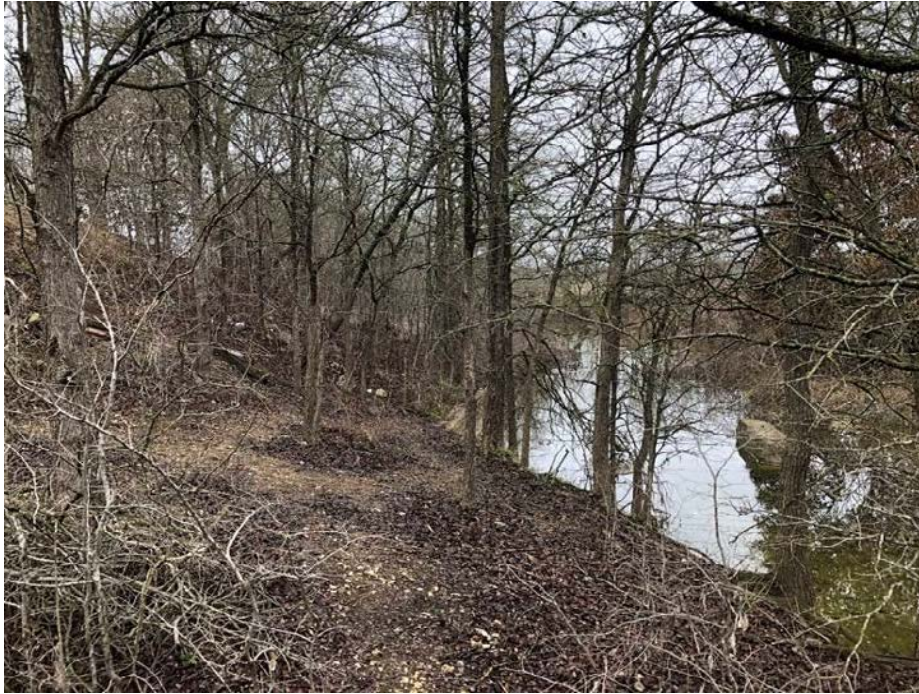
Figure 10. Site 41WM1435, remnants of the railroad bridge across Smith Branch Creek at the north bank of the creek, facing east. The northern railroad embankment is evident at the left side of frame. A concrete bridge abutment is evident at center of the frame. A remnant concrete bridge pier is evident in center of creek at the right side of frame.
