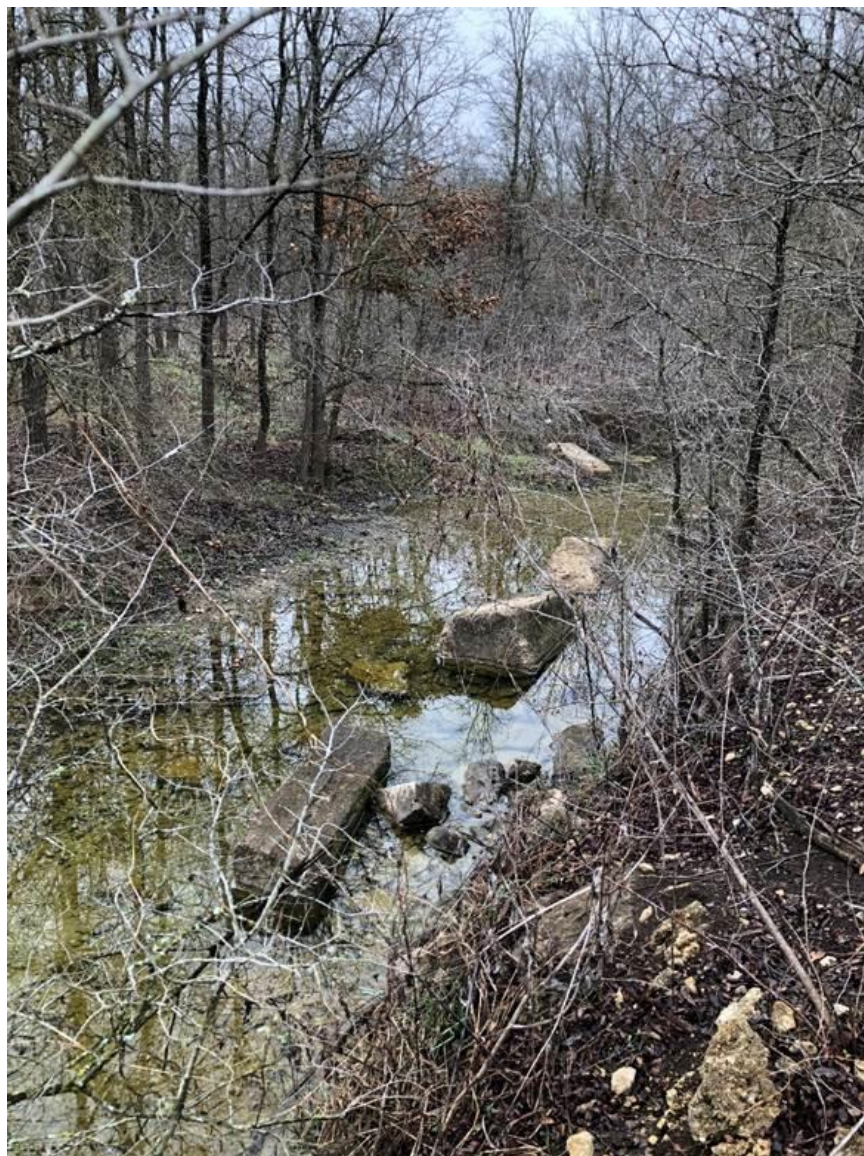
Figure 14. Site 41WM1435, disturbed concrete block remnants in Smith Branch Creek approximately 30 ft west of the railroad embankment, facing east/northeast. These remnants are believed to be from the bridge that carried the railroad over Smith Branch Creek, facing east/northeast.
