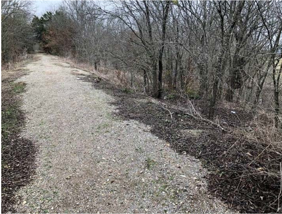
Figure 15. Site 41WM1435, railroad bed on top of the embankment approximately 250 ft north of Smith Branch Creek, facing south. Ballast is evident at surface.
