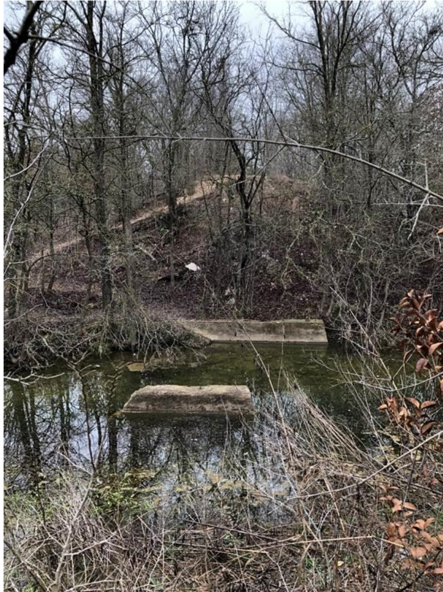
Figure 9. Site 41WM1435, remnants of the concrete railroad bridge substructure across Smith Branch Creek, facing north. Remains of the bridge are the concrete abutment and pier. Northern railroad embankment is evident beyond the creek at center with foot trail. Photo taken from top of railroad embankment at south bank of Smith Branch Creek.
