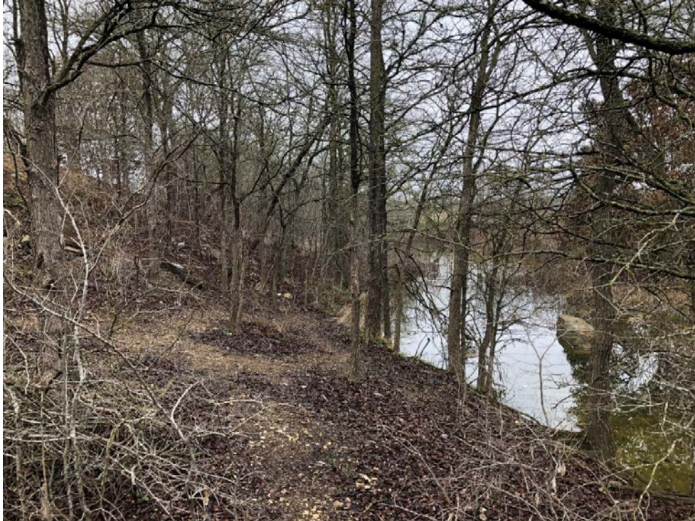
Figure 23. Site 41WM1435, remnants of the railroad bridge across Smith Branch Creek at the north bank of the creek, facing east. The northern railroad embankment is evident at the left side of frame. A concrete bridge abutment is evident at center of the frame. A remnant concrete bridge pier is evident in center of creek at the right side of frame.
