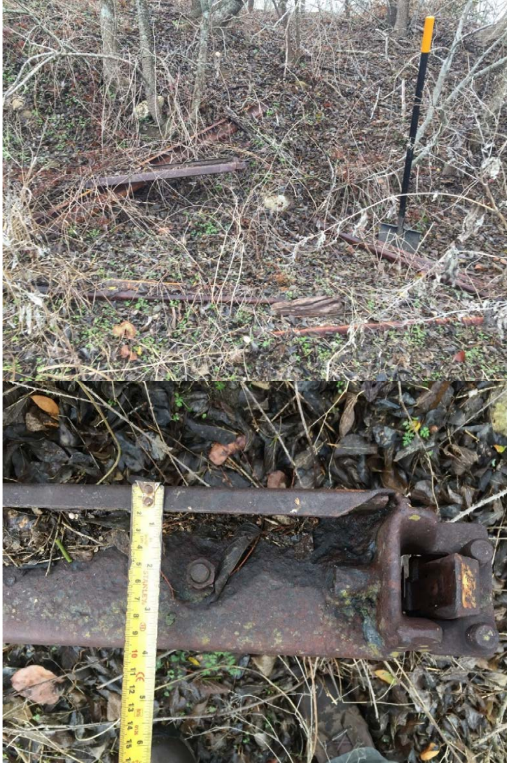
Figure 33. Site 41WM1435, Top-Group of possible fish plates on the upper east side of the railroad embankment, facing west. Bottom-Closer view of side of a possible fish plate. These remains are approximately 4 inches tall, with a flat foot and top that are 1 7/8 inches to 1 3/4 inches wide.
