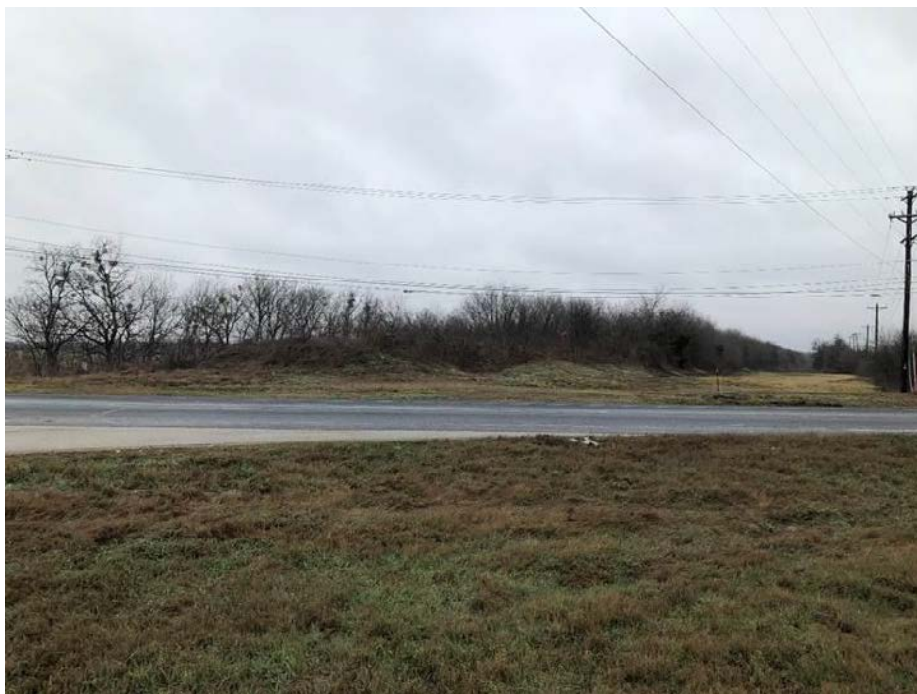
Figure 6. Site 41WM1435, overview of the MKT Railroad embankment that runs north through the APE, facing north. The embankment is evident as a raised earthen berm covered in vegetation. Southeast Inner Loop roadway is in foreground.
